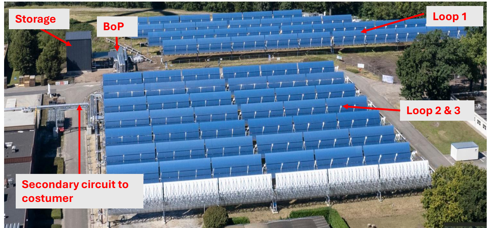
Solar collector field from Solarlite, Germany Power transfer station (BoP) and storage tank (Photo: Avery Dennison)
