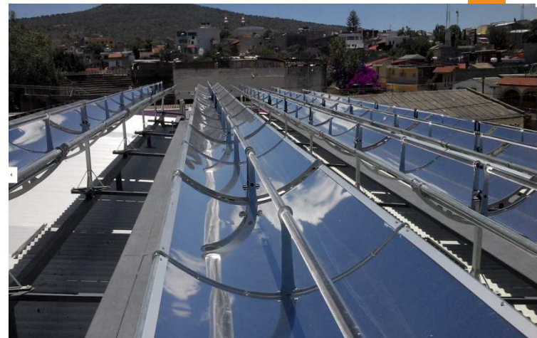
Dairy Plant – Mexico
